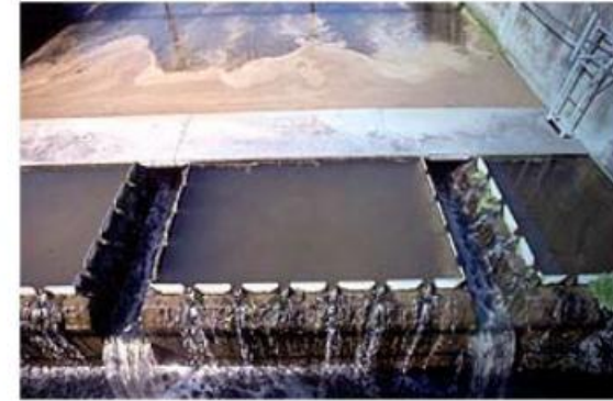
Activated sludge bed (left) and secondary settling tank (right) of WWTP Luzern
